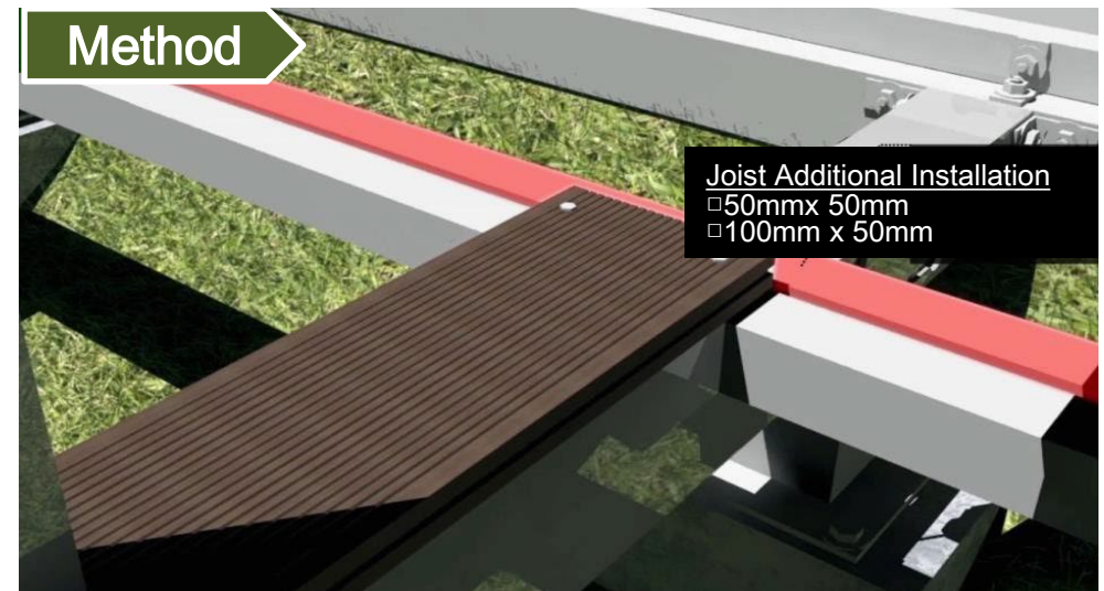
Screw position check (lengthwise 30mm, widthwise 20mm)
